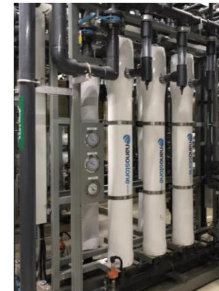
Grind WW (retrofit)
